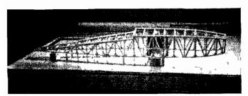
The top fuselage frame is then joined to the main fuselage section using 5/16" sq. balsa supports, reinforced with 1/32" plywood gussets.
